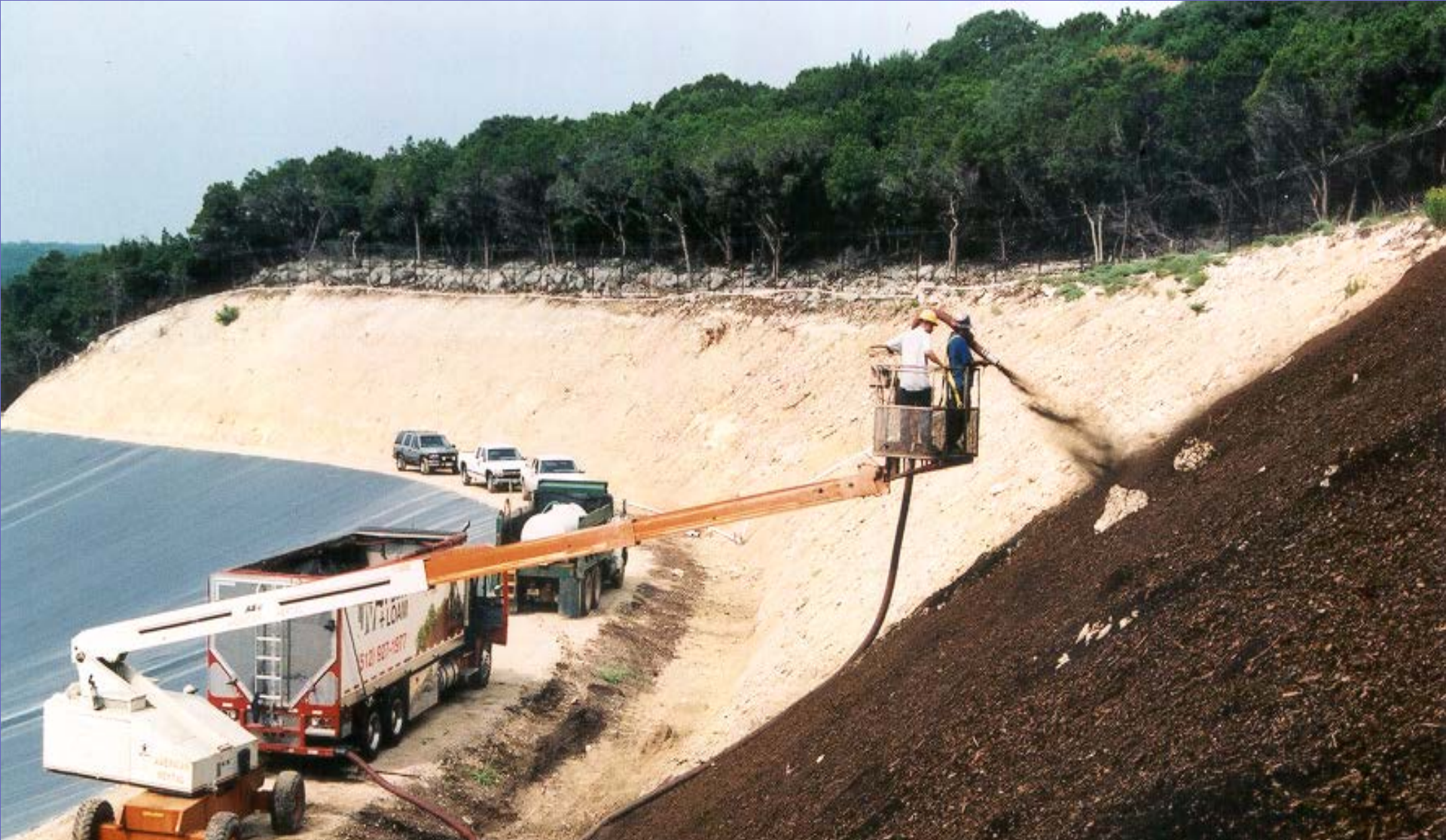
Application to 1:1 ROCK SLOPE 2" compost mulch w/native seed mix Barton Creek Development – Austin, TX AUGUST 17, 2002
